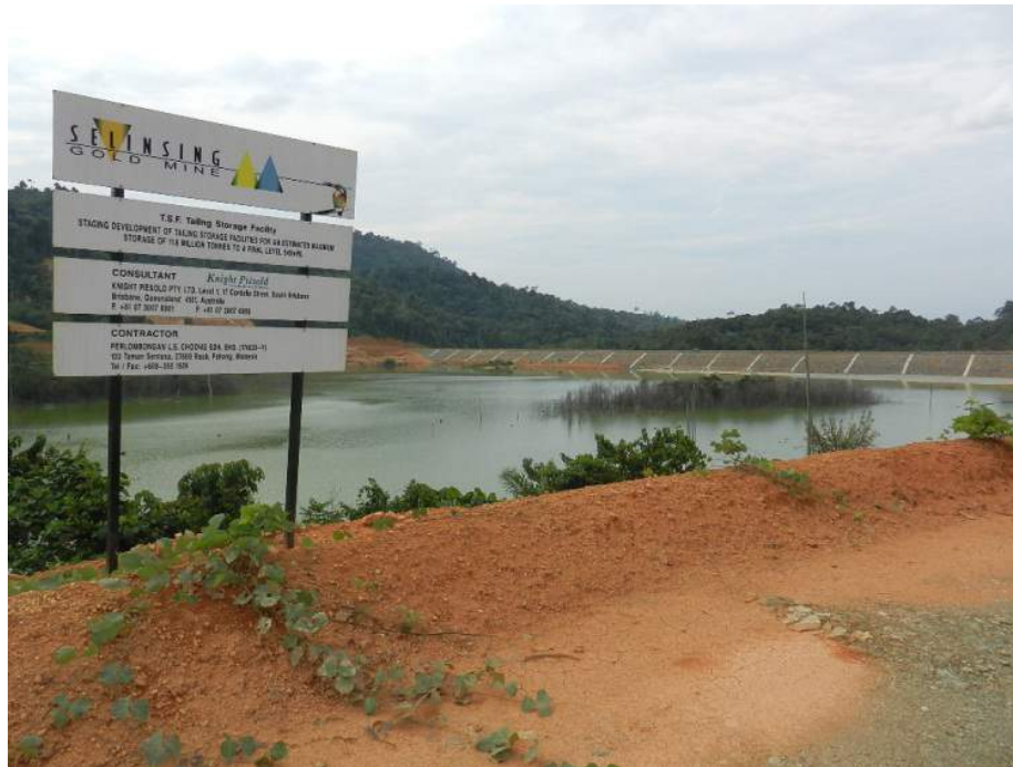
Figure 17.1.4 Selinsing Mine tailings dam and pond (June, 2012).
