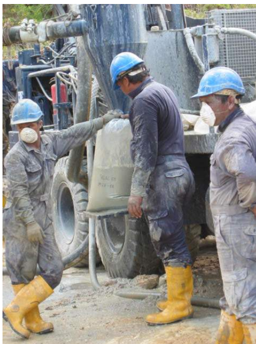
Figure 12.7 Collecting wet sample off cyclone
