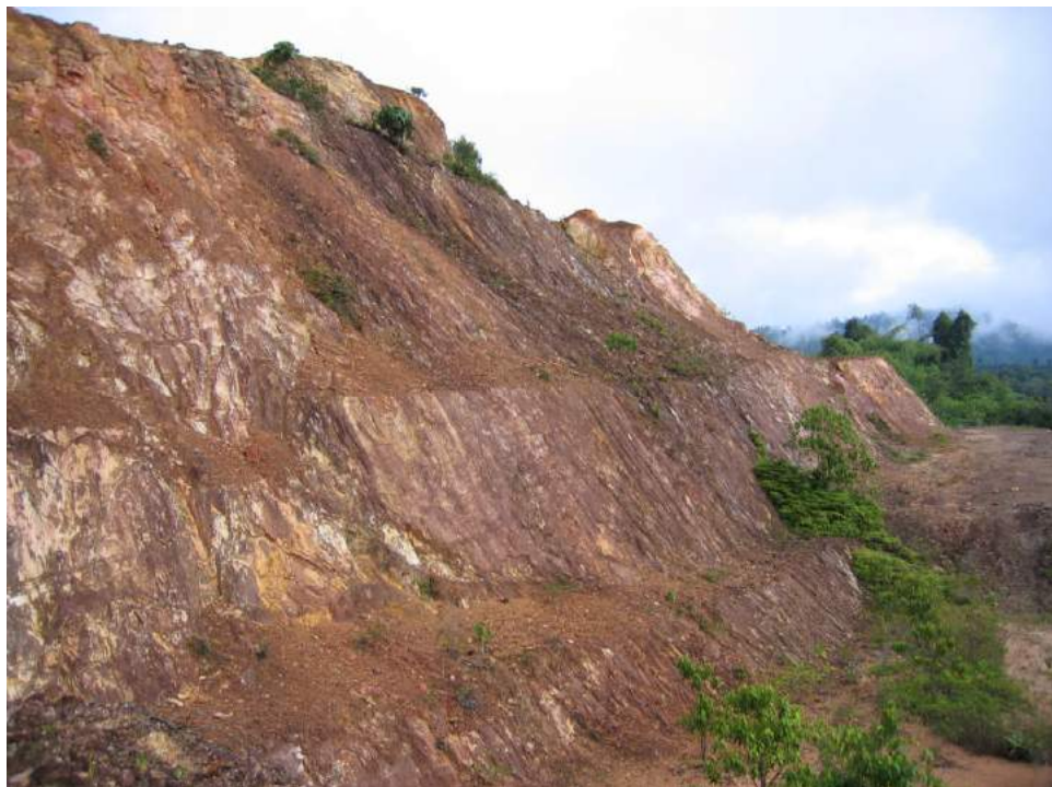
Figure 2.2 Current pit wall (west side)
