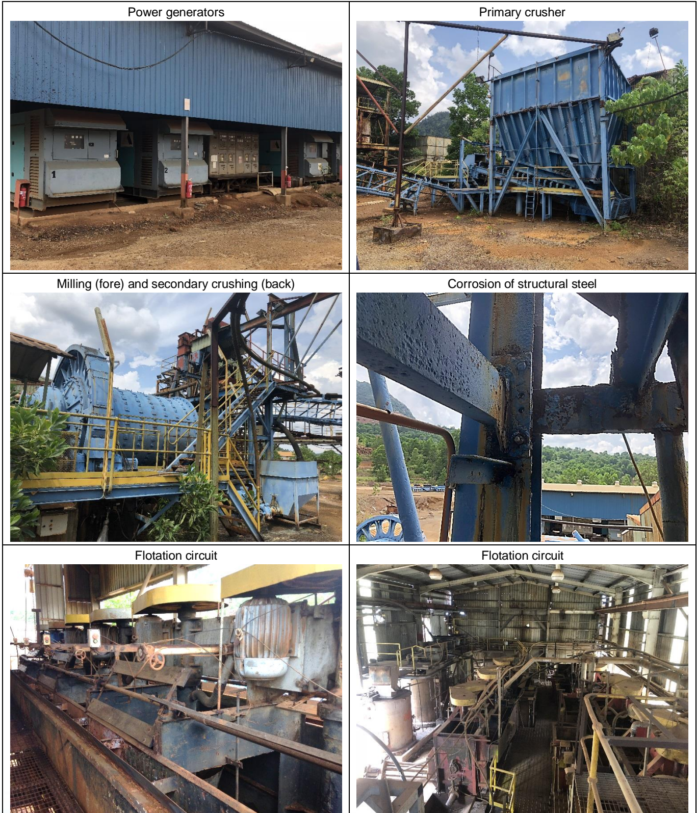
Figure 5.6 Photos of Mengapur plant and infrastructure taken during April 2018 site visit
