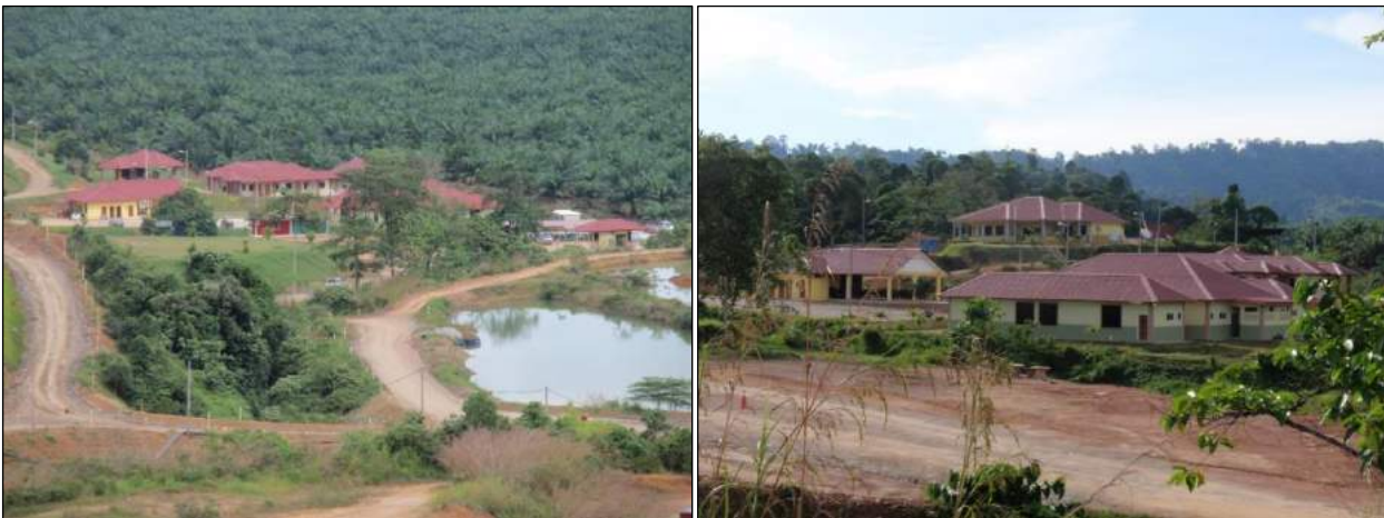
Figure 18.4 Accommodation and canteen complex (office is the building at the rear)
